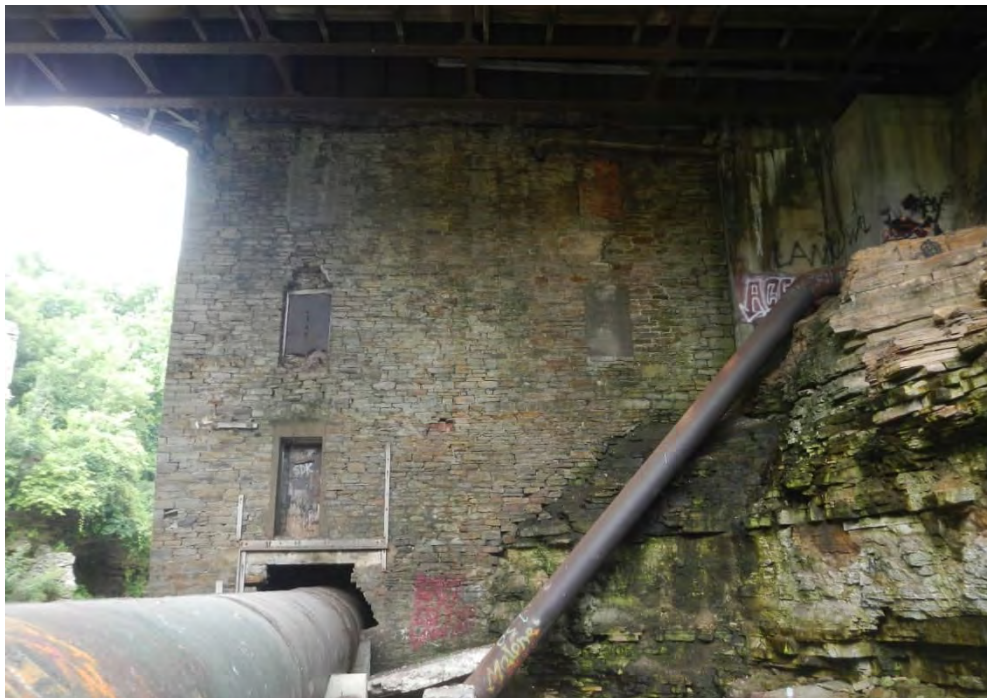
Photo 4-8 View of 399 Main Street building and Whittlesey dam penstock. US-11 bridge at top of image. The building significantly reduces the effective hydraulic opening of the bridge; note visible bulging of the structure along the left side.
