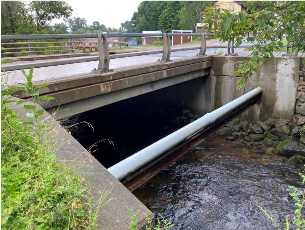
Photo 4-11 College Avenue crossing of Branch Brook, with utility crossing and supporting steel girder situated below the bridge low chord
