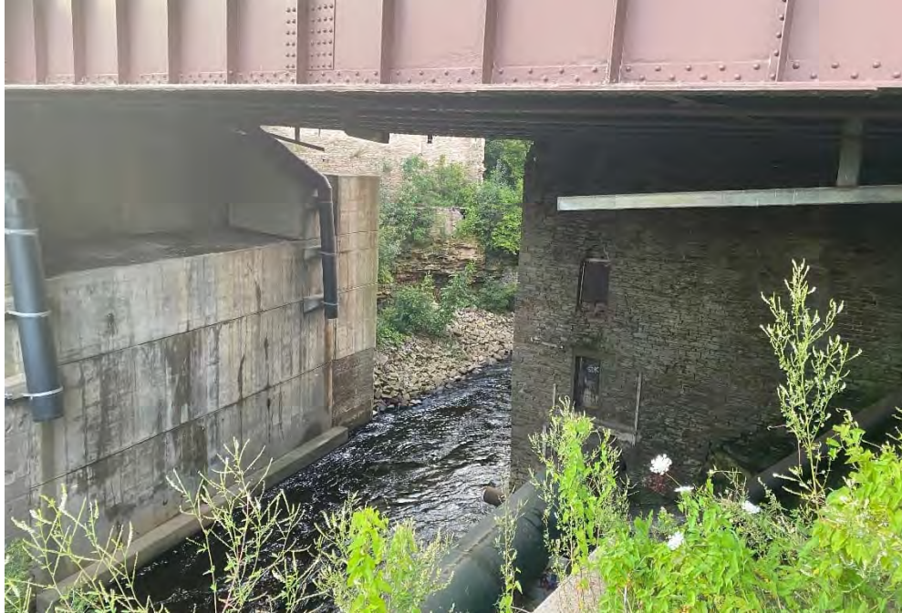
Photo 4-9 Whittlesey dam penstock entering powerhouse building beneath US-11 bridge, abutment at left. The majority of the bridge opening is obstructed.
