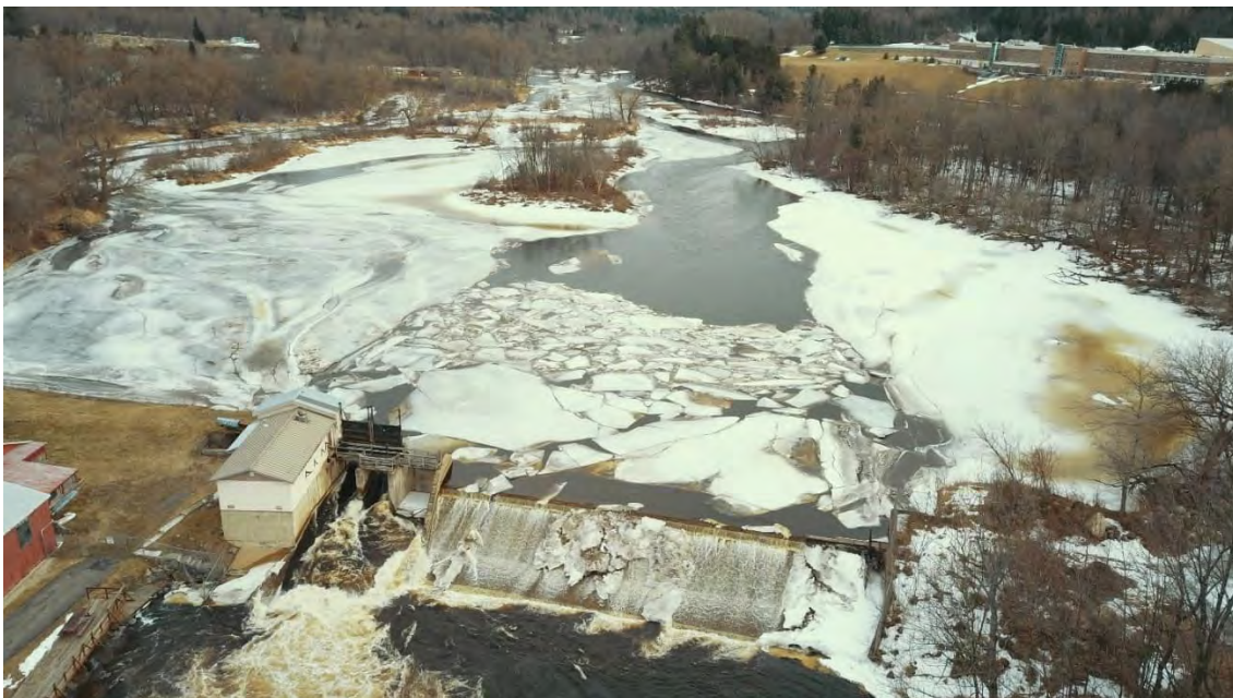
Photo 4-6 Ice formation and accumulation at Ballards dam. Photo provided by Village of Malone.
