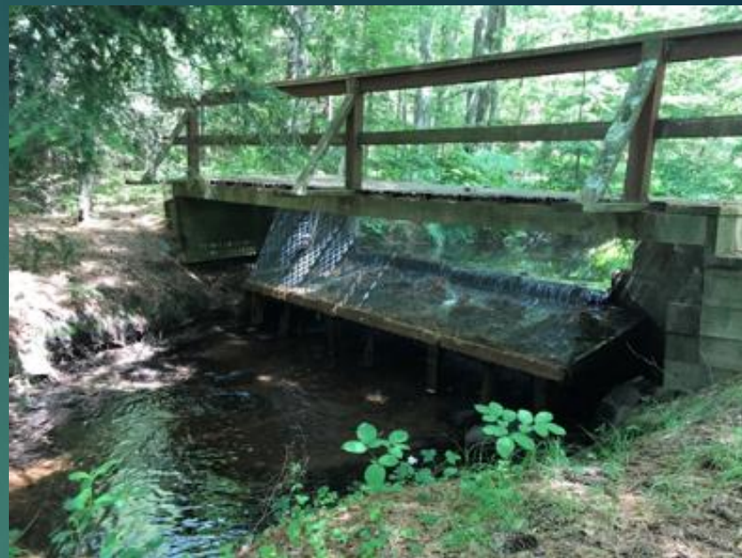
Fish Barrier Dam
