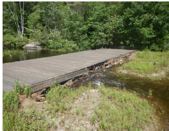
Hammond Pond Dam
