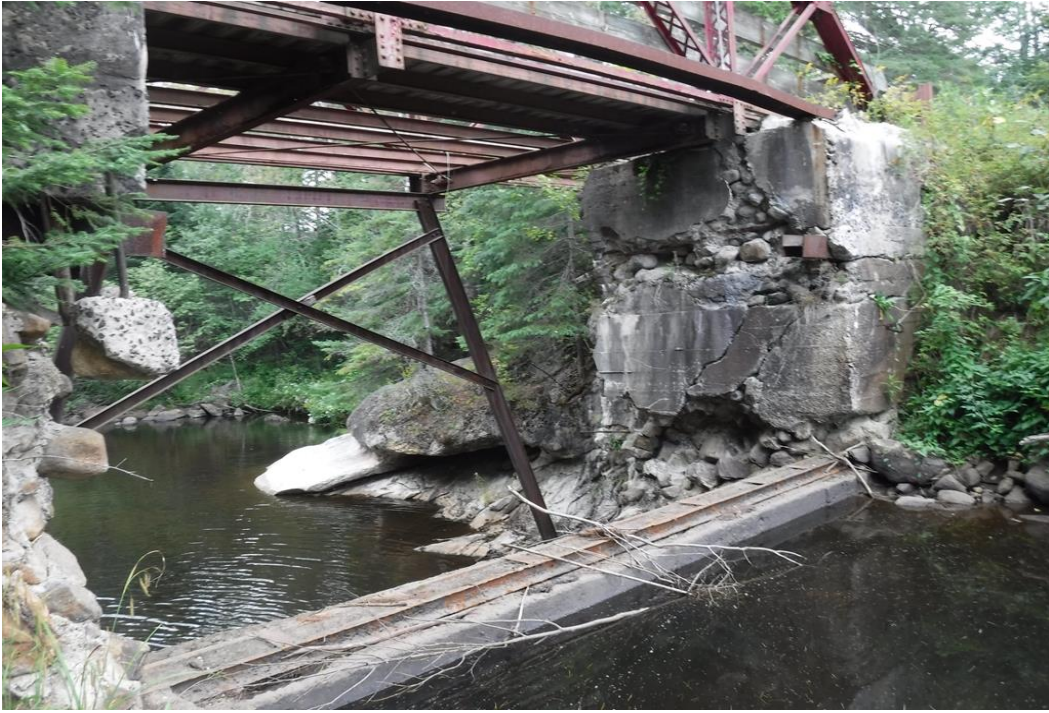
Photo 1 Dam ID# 186-0849 Rainbow Lake Dam 08/31/2018 Spillway looking downstream
