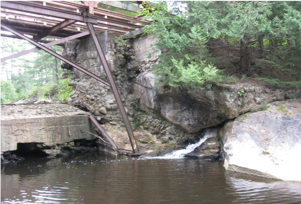
Photo 6 Dam ID# 186-0849 Rainbow Lake Dam 08/31/2018 Left downstream embankment
