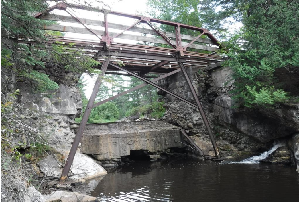
Photo 3 Dam ID# 186-0849 Rainbow Lake Dam 08/31/2018 Downstream view of the spillway
