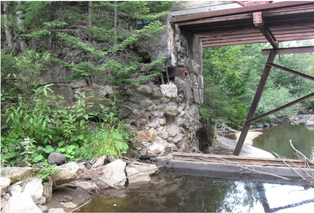
Photo 4 Dam ID# 186-0849 Rainbow Lake Dam 08/31/2018 Left concrete wall
