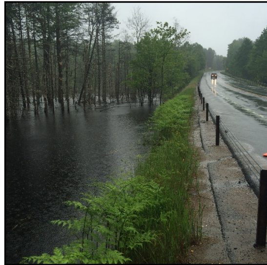
Figure 5.23 Beaver Impacts. Beavers have plugged a culvert forming a large water impoundment and creating a potential safety hazard.
