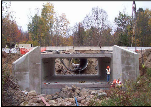
Figure 4.28 Box Culvert Replacement to Accommodate Aquatic Species Passage. During and after construction.
