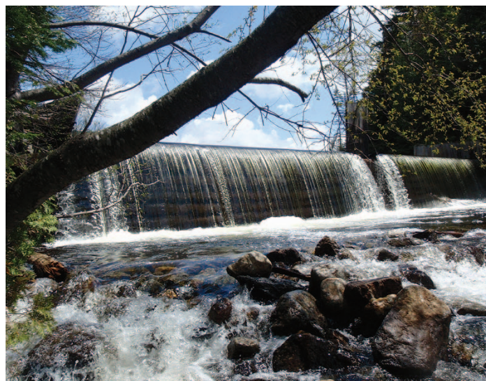
The Duck Hole dam was rebuilt in 1937.
